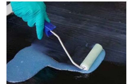
Roller application of SikaBiresin CR169 thix
