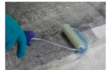
Wet lay-up with SikaBiresin CR168
