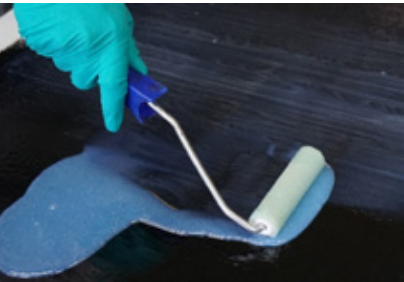
Roller application of SikaBiresin CR169 thix
